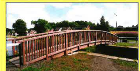
Footbridge supplied to British Waterways, at lock 14, Forth & Clyde Canal, Falkirk.
